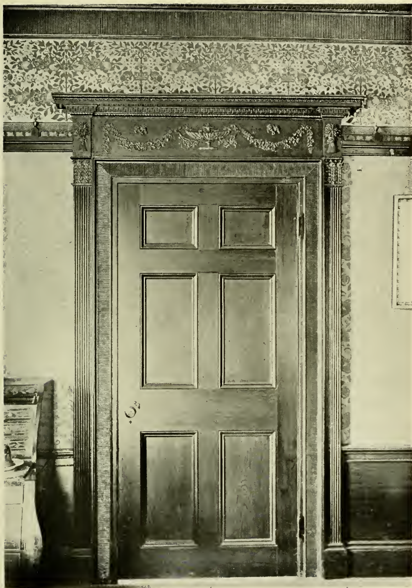
PLATE XXXVIII.—Doorway of the Morning Room, "Oak Hill."
